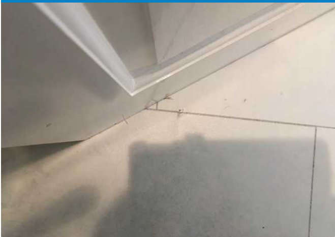
Small rip where door has jammed on it
